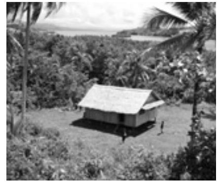
Atoifi Hospital, Kwaio.
